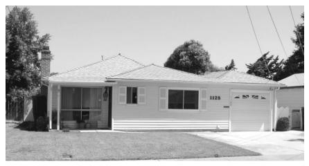
This house, in the same tract as the one shown above, has been extensively altered with a front addition, replacement of the original picture window, new façade windows on the addition, new siding, and a replacement garage door. It would be a non-contributor to an historic district.
