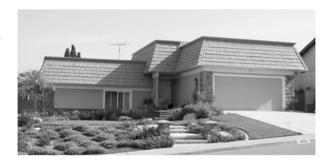
tilt-up type, and often clad in wood siding that matches that of the house. Builders began to use roll-up garage doors in the early 1970s. These are of wood, and can be easily distinguished from later, vinyl-clad roll-up garage doors. Aluminum sliding sash are common by this time, rather than the wood double-hung or metal casement windows of earlier postwar houses.
