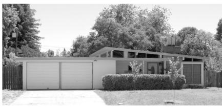
posts could be filled with glass or prefabricated, non-structural wall panels. The system made it easier to provide a much higher proportion of glazing to solid walls as compared to stud framing, where each window opening must be framed into the stud system.
