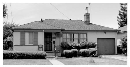
The windows to the right of the front door retain their original double-hung 2/2 wood sash, while the window to the left of the front door is a replacement sliding sash. With only this single alteration, the house could be a contributor to an historic district.
