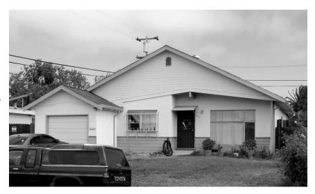
to houses constructed by builder Earl "Flat-top" Smith, either to reduce heat gain, shed rainwater more effectively, or simply give the house a more conventional appearance. Since the flat roof is the most distinguishing feature of Smith's houses, such alterations substantially diminish their integrity of design.
