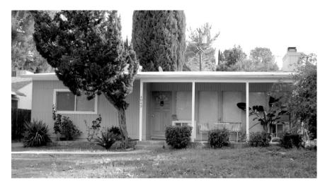
General Panel Corporation house in the San Fernando Valley of Los Angeles. Although the house has been extensively remodeled, the tall, narrow façade windows facing onto the front porch reveal the 40-inch panel width.
