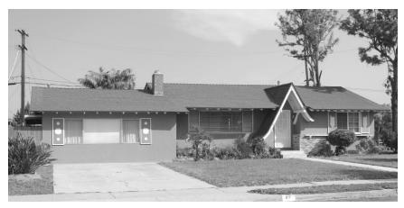
This house has new stucco on the walls, with a matching finish on the window trim, sills, and trim around the garage door. In addition, the windows, front door, and garage door are replacements. The house would be a non-contributor to an historic district, as its integrity of materials has been severely compromised.
