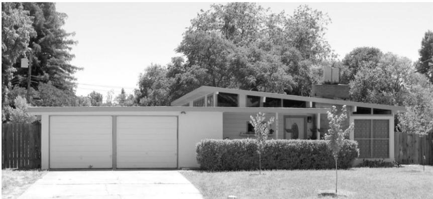
posts could be filled with glass or prefabricated, non-structural wall panels. The system made it easier to provide a much higher proportion of glazing to solid walls as compared to stud framing, where each window opening must be framed into the stud system.
