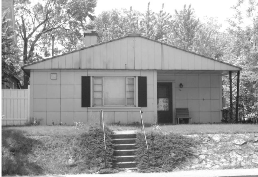
cabinetry, and even the roof shingles were also made of metal. The only visible materials on the inside or outside of a Lustron house that were not made of metal were the window glass, porcelain bathroom fixtures, and carpet or tile on the floors.
