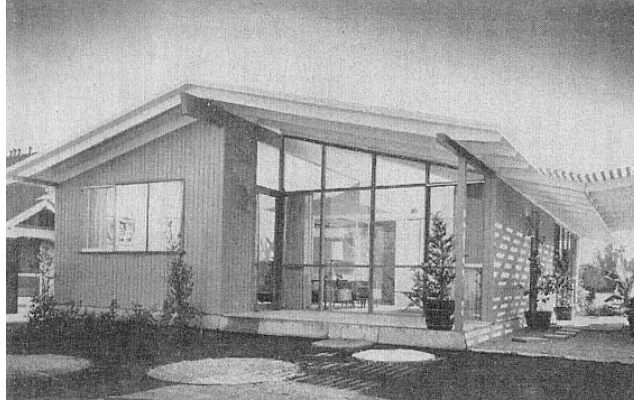
Figure 2:16 Rear elevation of McDonald Brothers design with wall of windows at rear. Channel-grooved wooden frames reduce time and materials associated with additional trim pieces for glass. "House Designed to Be Trucked to Site," House and Home , June 1956, 148. Photo by George de Gennaro. Permission pending.
