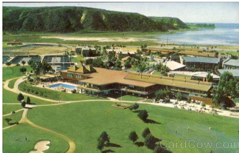
Figure 2:28 La Costa postcard shows T-shaped plan of the clubhouse with skylights on spine of long gabled roof form at right. Used with permission of La Costa Resort and Spa. http://www.cardcow.com/105405/rancho-la-costa-carlsbad-california/
