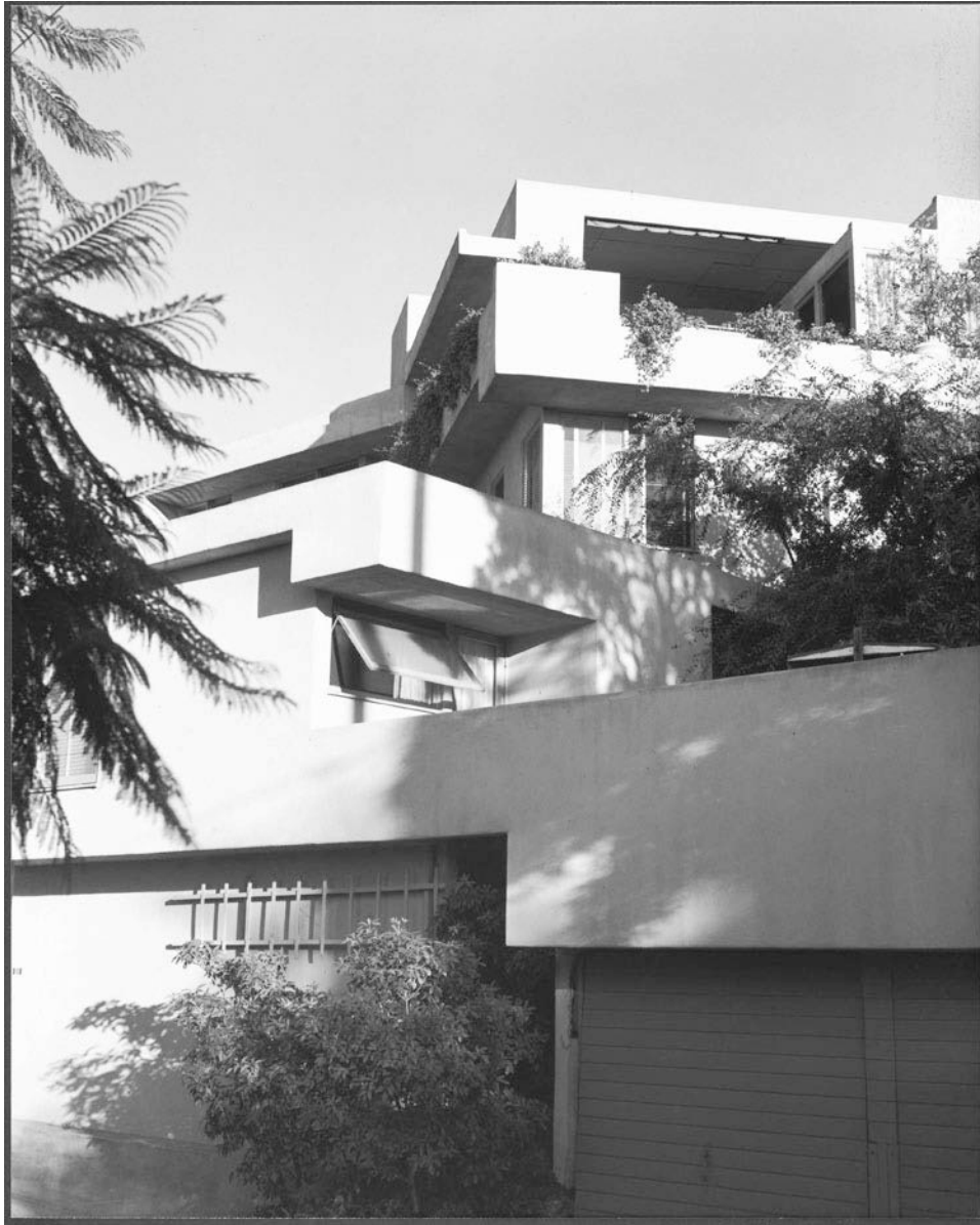
Figure 4:4 Falk Apartments (1939-1940) by R.M. Schindler. Copyright: © J. Paul Getty Trust. Used with permission. Julius Shulman Photography Archive, Research Library at the Getty Research Institute (2004.R.10).
