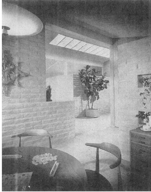
Figure 2:22 Post-and-beam construction offered Fickett an open plan in this tract house for Elwain Steinkamp. Skylights for control of natural light and rustic materials enhance the design. "Quality Houses at $10.50 a Square Foot Win NAHB Award," House and Home , March 1955, 160. Photo by George de Gennaro. Permission pending.
