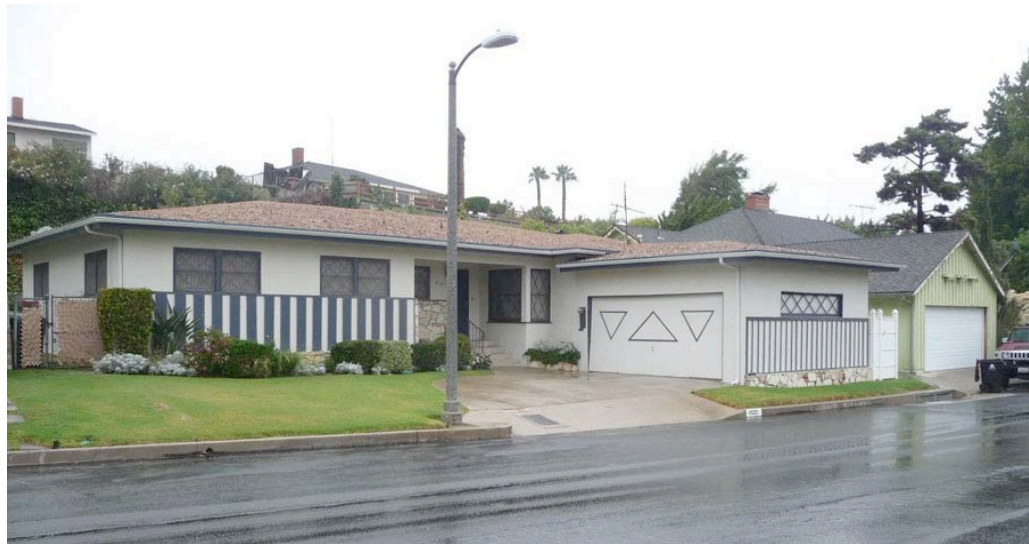
Figure I:5 Example Ranch Contemporary house. Baldwin Hills Estates tract (1950-59). Used with permission. Copyright ARG/SurveyLA 2010. Not for reproduction.
