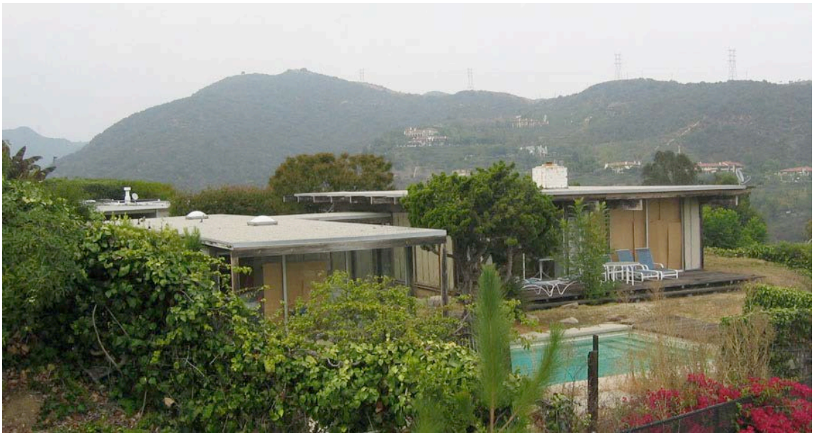
Figure I:6 An example of post-and-beam construction clearly visible in the post-and-beam aesthetic. Mullikin Residence (1964) by Richard L. Dorman. Photo by the author.
