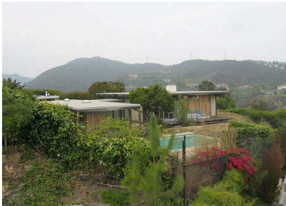
Figure 3:14 Mullikin Residence (1964) features the post-and-beam aesthetic. The house is currently in disrepair with its vast expanses of glass covered by cardboard. Photo by the author.
