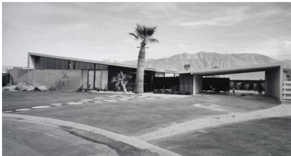
Figure 4:21 Example of butterfly roof design used extensively in the Palm Springs developments for George Alexander. Copyright: © J. Paul Getty Trust. Used with permission. Julius Shulman Photography Archive, Research Library at the Getty Research Institute (2004.R.10).
