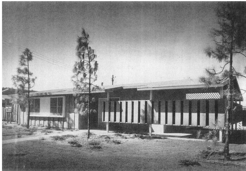
Figure 2:13 Elevation for "Plan A" at Sherman Park in Reseda. Articulated screen gives elevation length and hides carport. Style is clean, contemporary ranch. "The Fickett Formula," House and Home , March 1953, 134. Photo by Julius Shulman. Copyright: © J. Paul Getty Trust. Julius Shulman Photography Archive, Research Library at the Getty Research Institute (2004.R.10). Permission pending.
