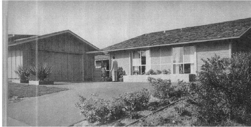
Figure 2:19 Board and batten walls, roof shakes, and masonry planter are examples of rustic materials used by Fickett in this design for Walter R. Sant and Sons in Palos Verdes. "Modern Design Can Create A Nostalgic Setting," House and Home , October 1955, 172. George de Gennaro. Permission pending.
