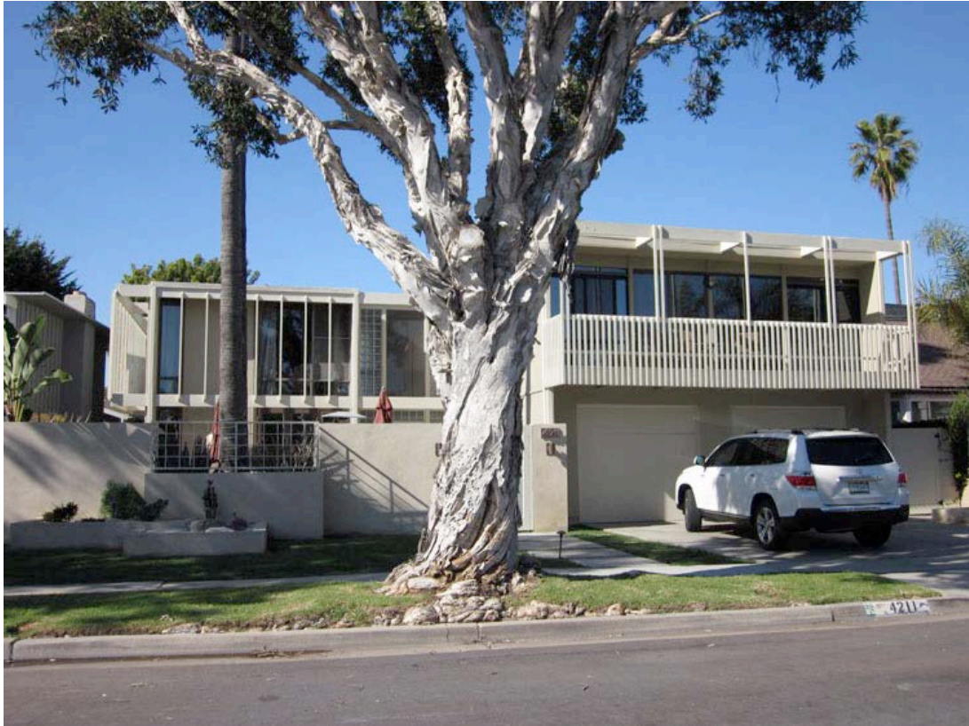
Figure 3:7 Dorman’s flat-roofed modern tract home from the Huntington Harbour 1965 Series with significant alterations, including second story garage addition, altered wooden screen fenestration and entry wall. Most all other models constructed have been razed or remodeled beyond recognition. Photo by the author.
