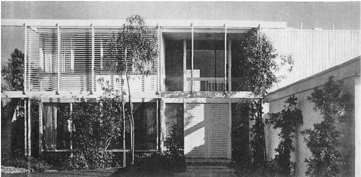
Figure 3:6 Richard Dorman's two-story flat-roofed model home for the 1965 Series at Huntington Harbour featured simple, rectangular form with central sculptural stairway visible through large panes of glass. Wooden lattice screens provide shade and privacy on front elevation. Photo by Richard Gross. "A Two-Story Contemporary That Stresses Openness," House and Home , March 1966, 106. Permission pending.
