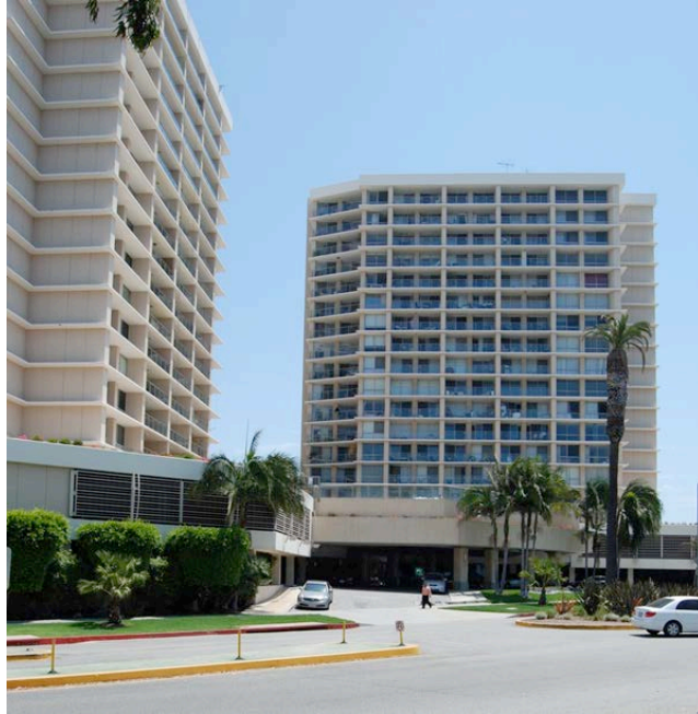
Figure 4:34 Front elevation of Ocean Towers (1971) by Krisel/Shapiro shows how towers have been angled for maximum views and shared public areas. Photo by John Berley.
