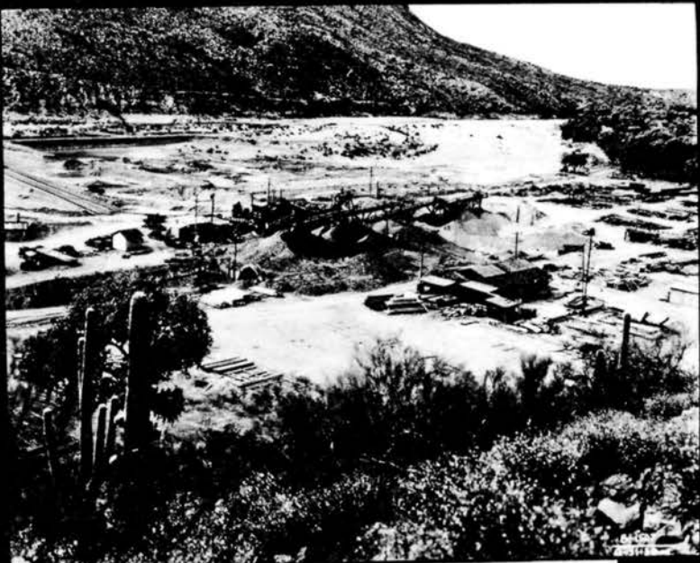
BARTLETT DAM: B-1807, View of aggregate processing plant and aggregate deposit. -P.
